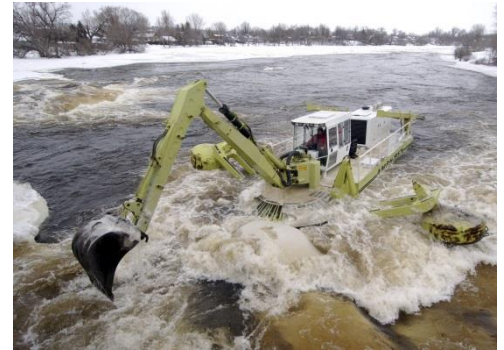
Ice breaking in North America with Amphibex excavator (Normrock Industries Inc.)
